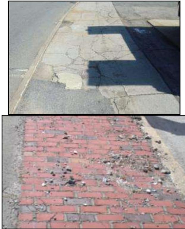
**Figure 5: Cracked Sidewalk (left); Poorly maintained brick (right)**
