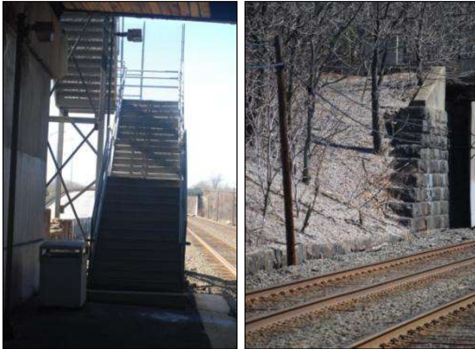
Figure 4: Inaccessible Commuter Rail Station
