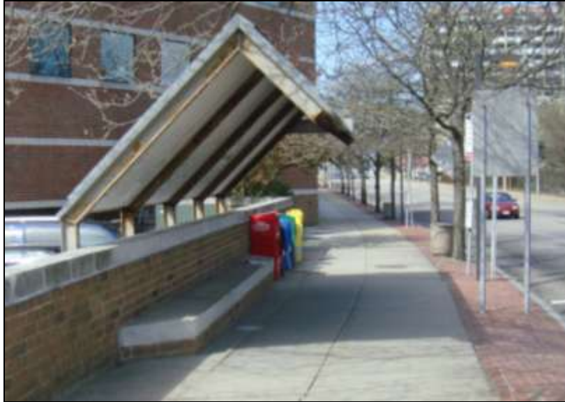
Figure 4: Newton Corner south bus stop
