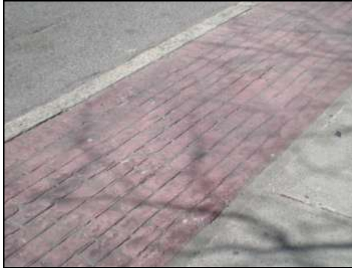
Figure 3: Pressed concrete on Washington Street in Newton Corner
