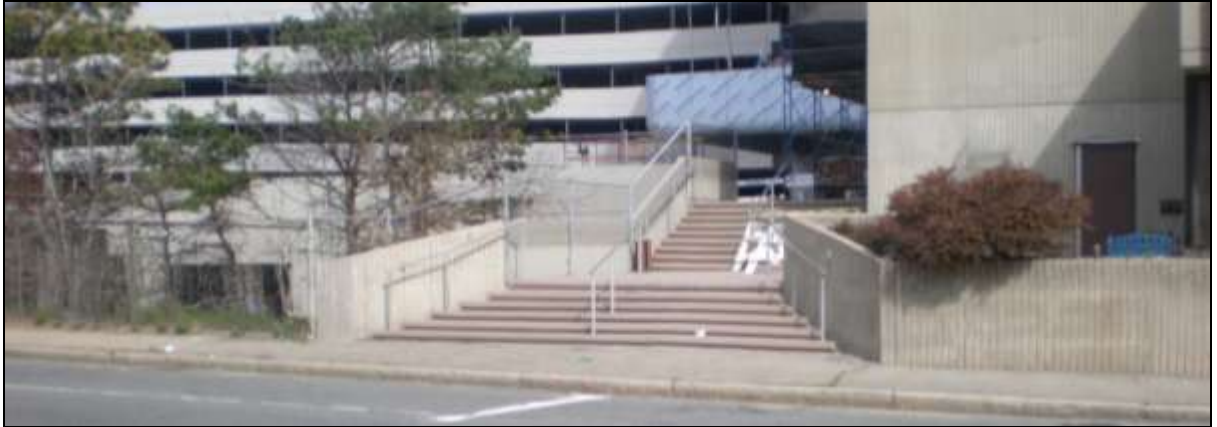
Figure 7: Crowne Plaza path - south side
