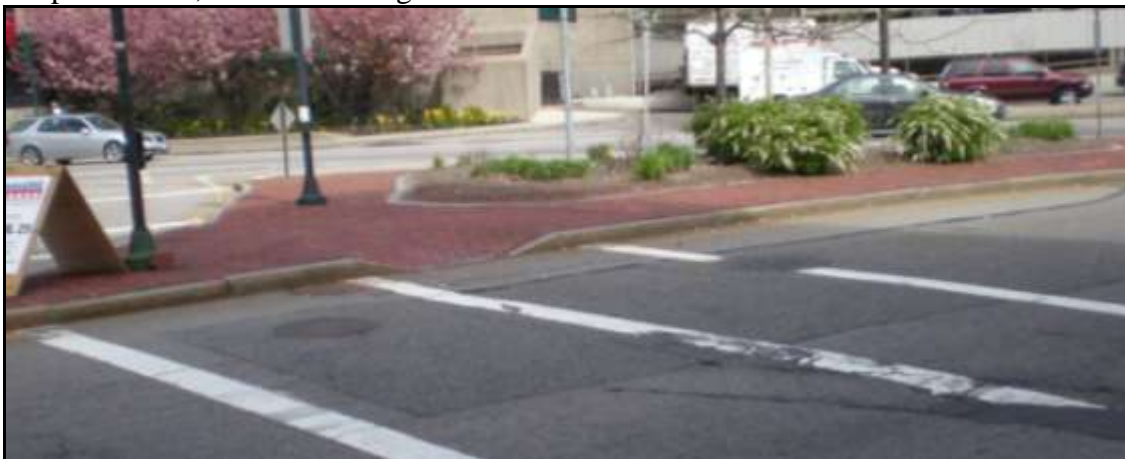
Figure 9: Median at Centre Street and Centre Avenue
